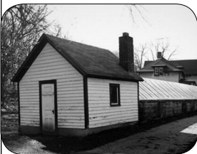
Green house at Tyrawley
